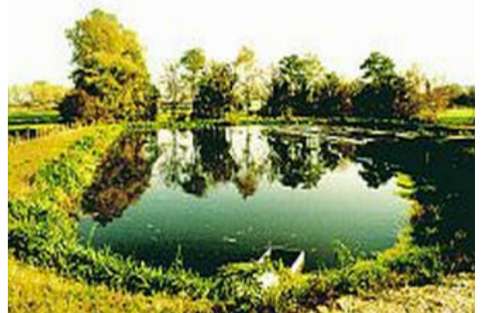
Advanced Wastewater Pond
