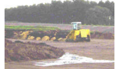
Solar Sewage Sludge Treatment, EU
